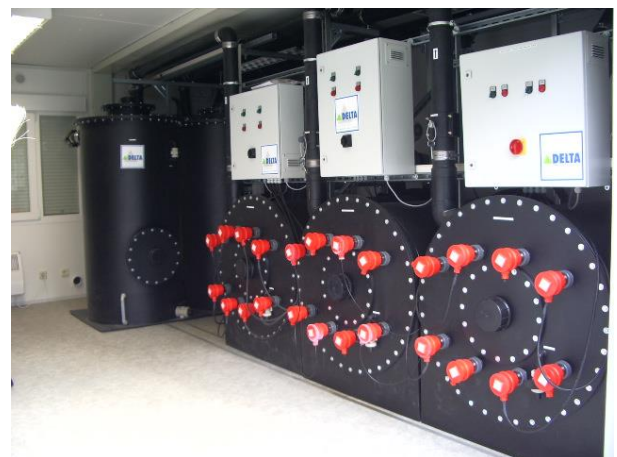
Photolysis reactor for ground water treatment
